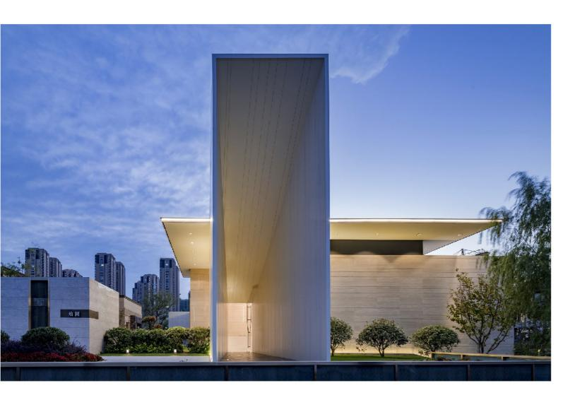
Environmental friendly material is applied in all the spaces of the building. Steel structure is used for architectural structure and frameless glass curtain wall is designed to connect the exterior and the interior space. Façade of the building is applied with calcium silicate board which is a kind of cost-efficient material and can be installed easily with compliance to relevant water-proof and fire-proof codes.
